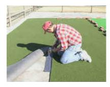
**For Foam Backed Turfs:** Do not cut a straight line in a turf with a foam backing for seaming, because you cannot see the rows of stitching. If you want to seam sections together yourself, ask us to true-cut the sections at the factory so that the seams will fit together correctly.
